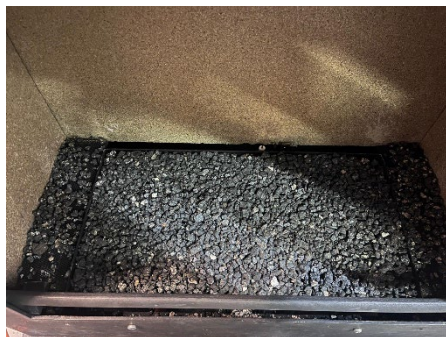
Fig.11 Add vermiculite to mesh trims
