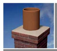
Commonly in older houses, earlier than 1960. The Class 1 chimney is identifiable by 7" (180mm) or greater diameter flue. The existing chimney must be structurally sound, please check before the installation of a new fireplace.
