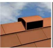
Modern houses generally later than 1960 often have a precast concrete chimney system, identifiable by a rectangular box section flue and a terminal, as illustrated in the picture above
